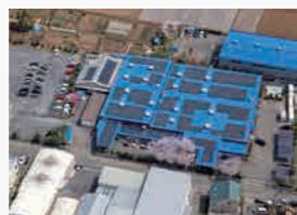
Factory rooftop, SHINANO INC.
